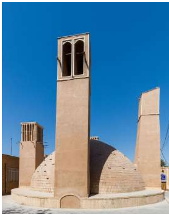
Fig. 3. An water reservoir (ab anbar) with double domes and wind catchers (openings near the top of the towers) in the central desert city of Yazd, Iran, [6]
